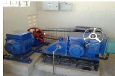
Gambar 6. Model Turbin *Cross Flow*
