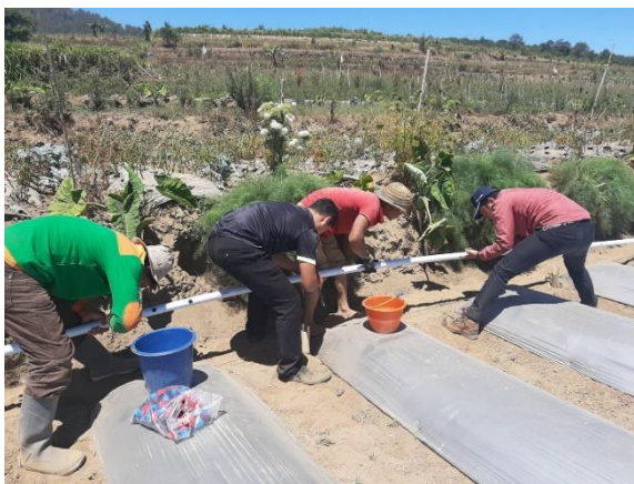
Gambar 6. Instalasi Jaringan Pipa Manifold
