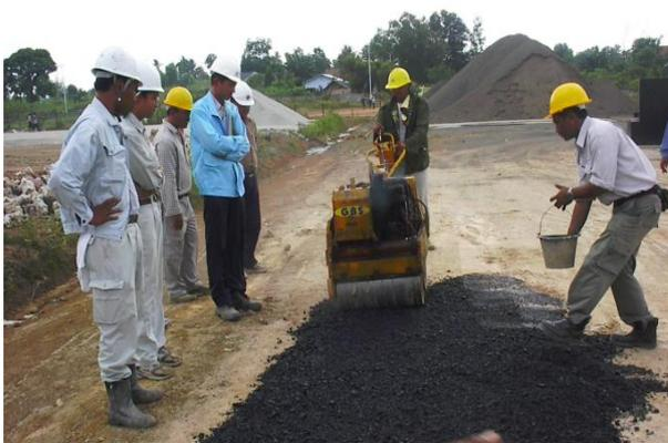
Gambar 9. Trial Mix Terhadap Lapis Bituminous
