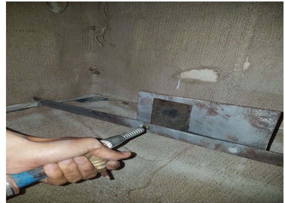
Gambar 2. Proses Sandblasting
